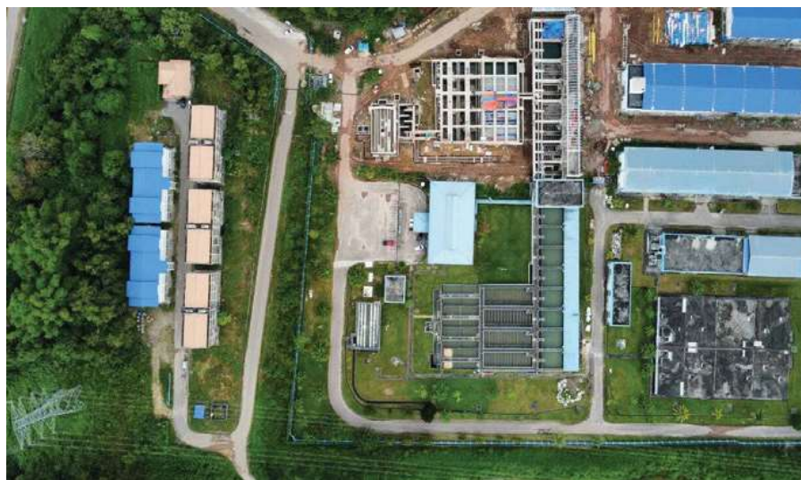
Aerial view of Telibong water treatment plant
