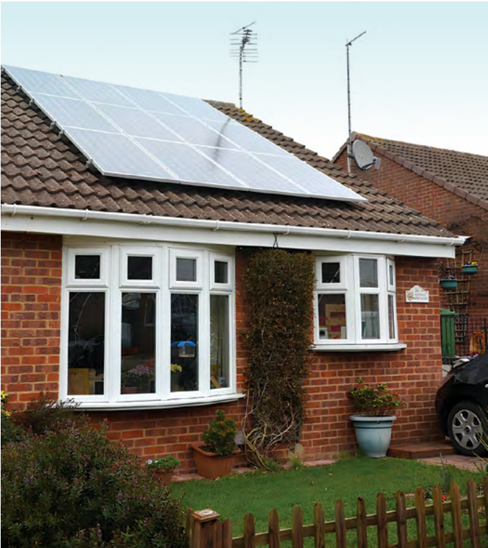
Residential solar rooftop installation in Northampton
