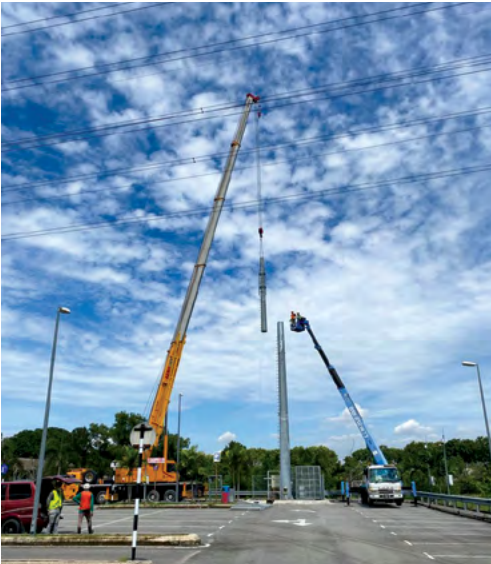
Relocation of 30m pole at Subang Alam
