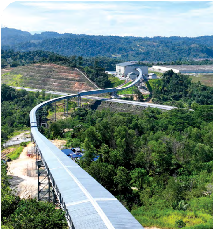
Overview part of sludge conveyor
