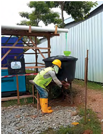
Rainwater harvesting system installed at Kuala Kubu project site to reduce reliance on conventional water sources
