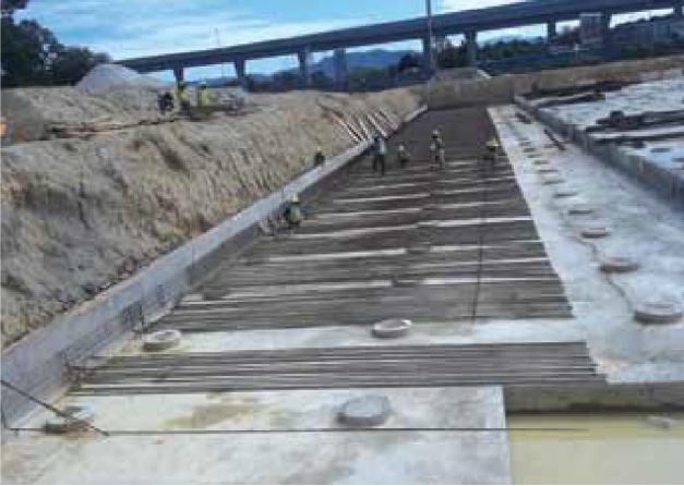
Primary Clarifier Piling & Lean Concrete works at Langat CSTP project site.
