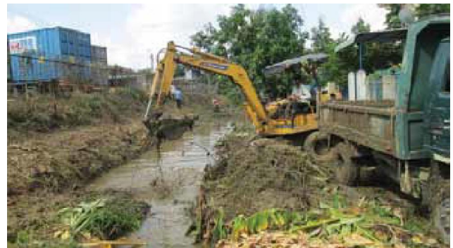
BAWC JV with Binh Thang People's Committee cleaning external drainage.
