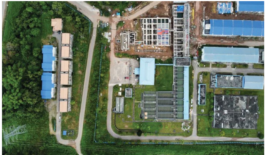
Aerial view of Telibong water treatment plant
